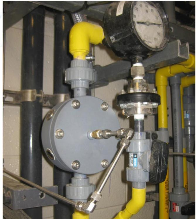
*Close up of 3/4" CPVC Equilibar back pressure regulator in Sodium Hypochlorite service.*
